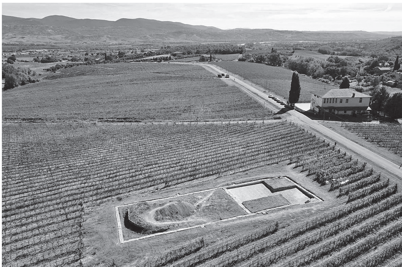
Fig. 2. Aerial view of the cistern at Spoletino, from west.
