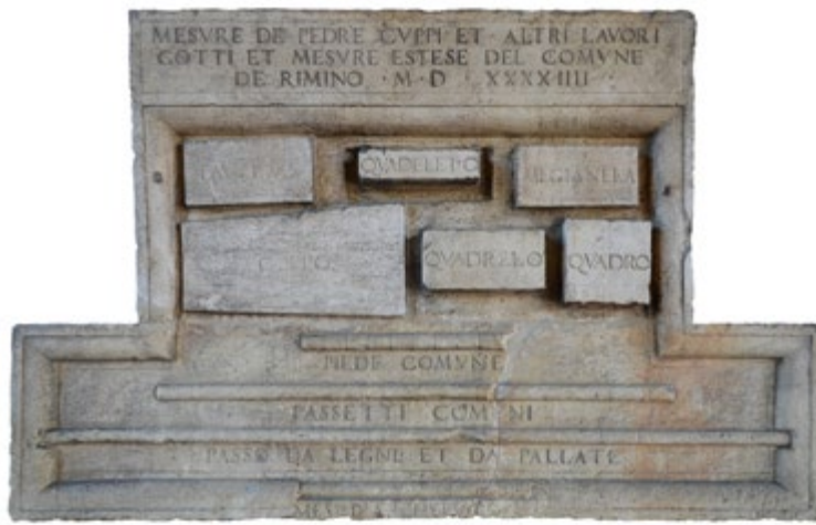
Fig. 5. Abacus with the local units of measure and the fixed dimensions for some building materials, 1544. Rimini, Loggia of Palazzo dell'Arengo (from Fiorini 2015, 82, fig. 6).
