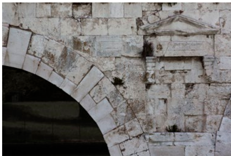
Fig. 17. Bridge of Augustus and Tiberius. A detail of the external wall casing. The lighter color ashlar are evidently the ones that were restored and have the mark of R 1976.
