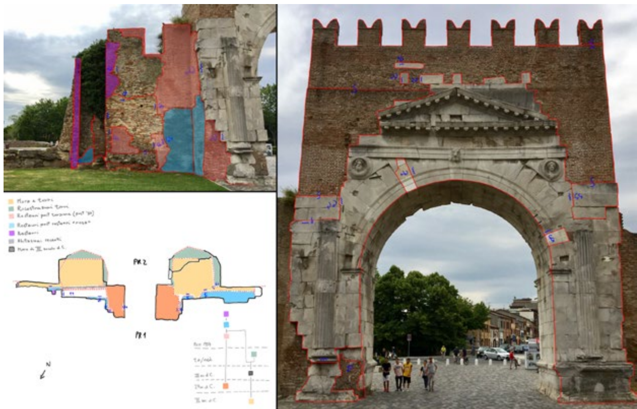
Fig. 10. Arch of Augustus. Stratigraphic annotations recorded in the field using a PC tablet.
