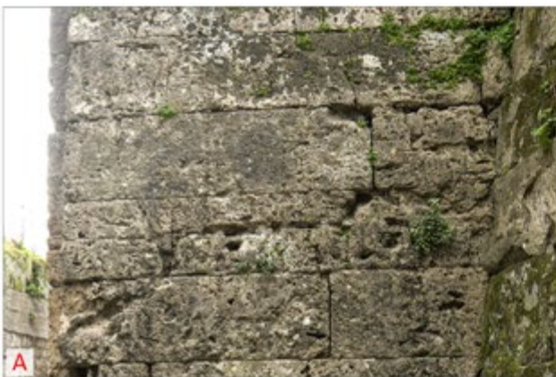
Fig. 11. Evaluation of the intensity of the phenomenon of biological colonization on the stone surface. Image A: Wall surface of the Left Bastion of Porta Nola. Image B: wall surface of the section between Porta Nola and the left Bastion
